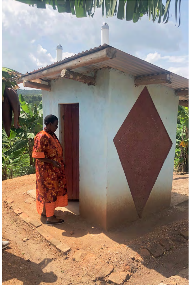
Safe toilet construction in Fort Portal, Uganda. ©Eike de Buhr/SHF
